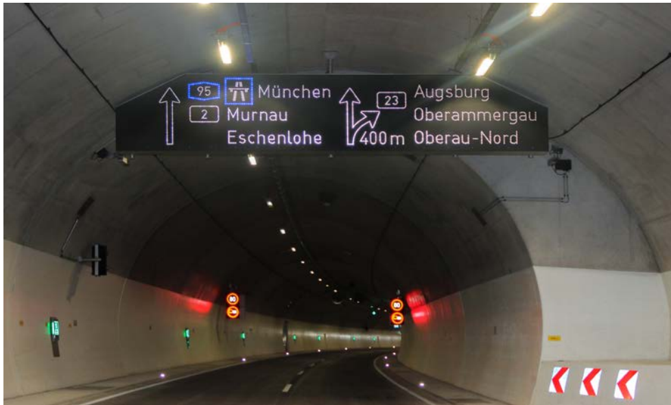
The slanted LED-type exit indicator is a special design to match the location's geometry.
