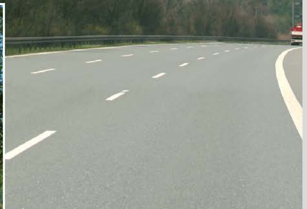
BAB A73 Motorway at Nuremberg, Germany
