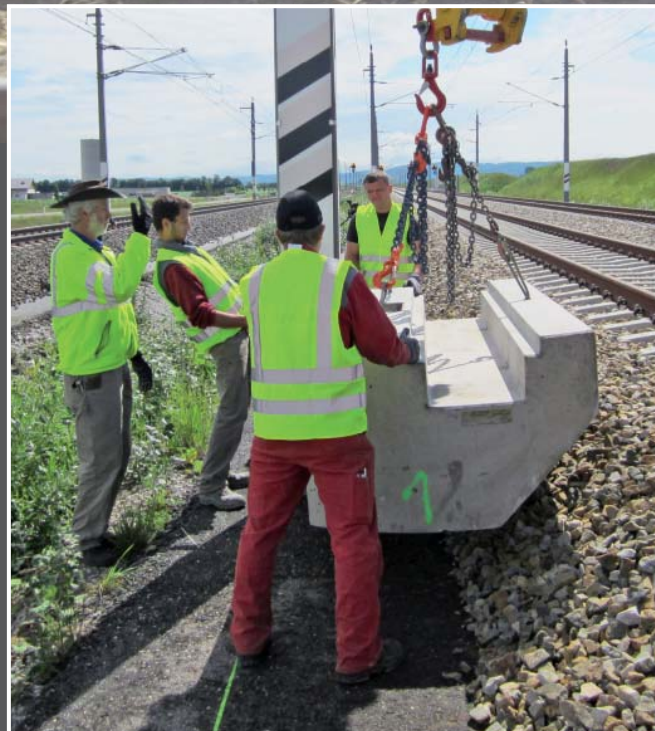
Setting of the concrete base
