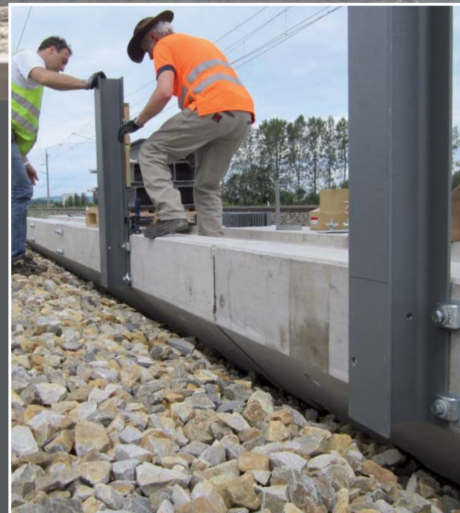
Installation of the posts
